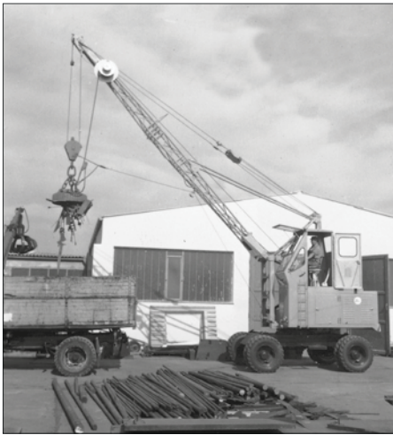
1962: rope-driven S833 with elevated operator cab
