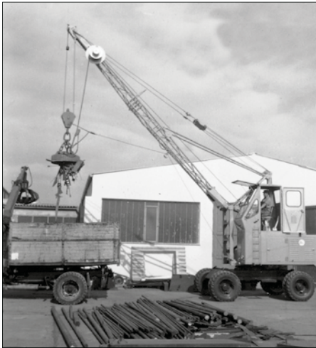
1962: rope-driven S833 with elevated operator cab
