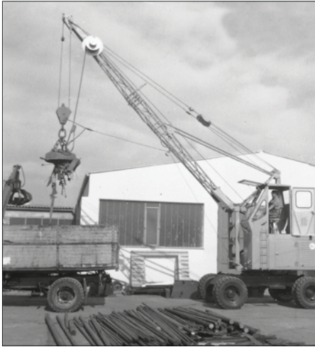
1962: Rope-driven S833 with elevated operator cab
