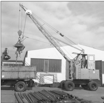
1962: rope-driven S833 with elevated operator cab
